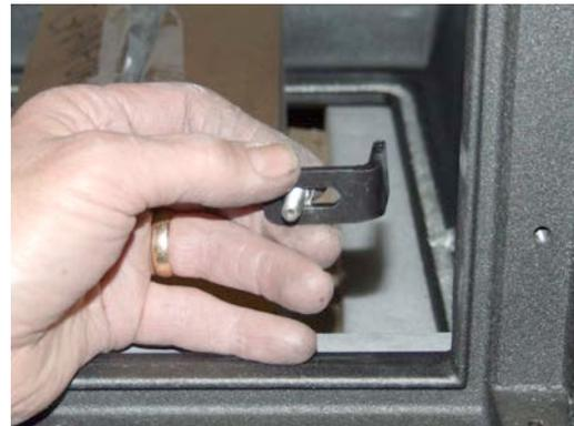
13. It will be necessary to mark the draw rods with a black marker to ensure they are set at the proper depth in the top cast iron frame. Mark the face of the rod and
