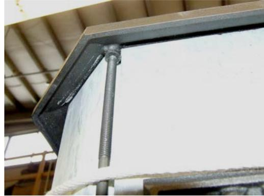
14. Install the cast iron corners. Slide the tops under the rope and swing the bottoms into place on the base of the stove.
