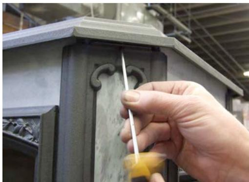
4. Tie a rope or strap around the body of the stove. The rope will hold the corner stones in place when the cast iron corners are removed. The rope should have enough play to remove the cast iron corners.
